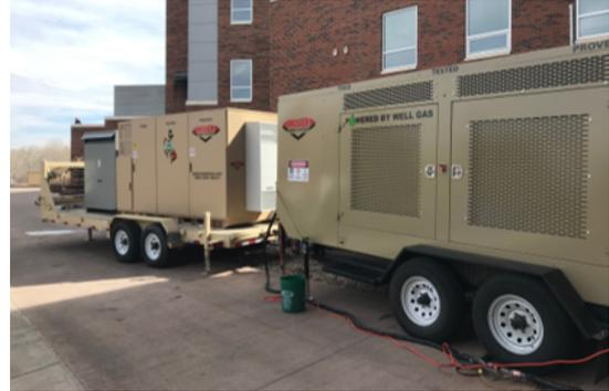
(b) NG-hybrid 11 L generator system with ESM trailer (left) and transformer (right).
